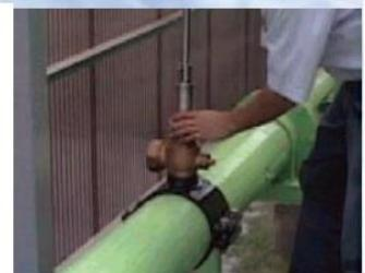
④Installation insert the flow meter
