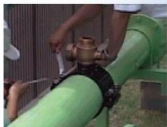
①The saddle points hydrant fixed on a pipe
