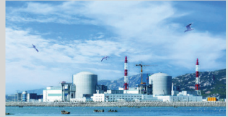
TIANWAN & QINSHAN NUCLEAR POWER STATIONS CHINA
